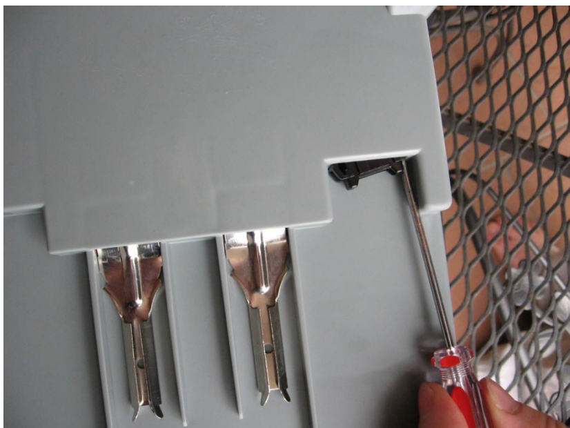
Picture: Unlocking and removing the fuse holder
